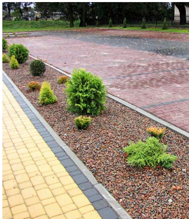
The parking in Czarna realized within "Renewal and rural development"
